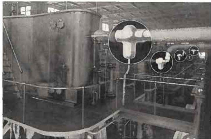
Six Type "E" Horizontal Live Steam Separators in Cleveland City Water Works, Cleveland, Ohio
