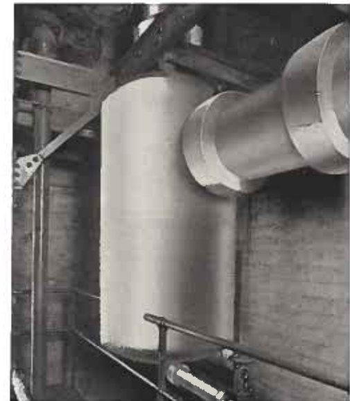
12" Angle Separator Under 275 Lb. Pressure 200° F. Superheat—Side Inlet and Top Outlet
