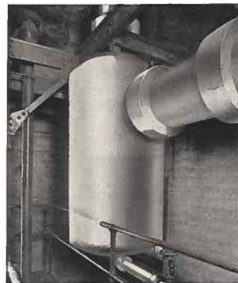
12" Angle Separator Under 275 Lb. Pressure 200° F. Superheat—Side Inlet and Top Outlet
