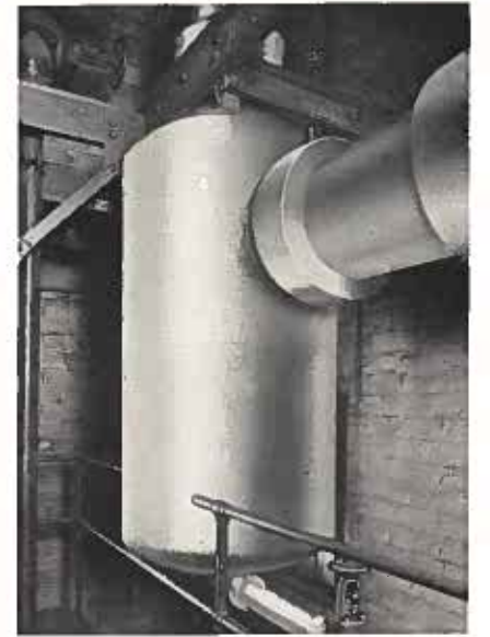
12" Angle Separator under 275 psi and 200° F Superheat. Side Inlet and Top Outlet.
